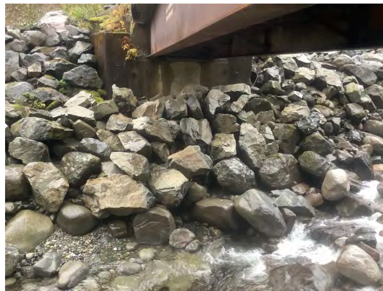
Right Bank Abutment when facing downstream
