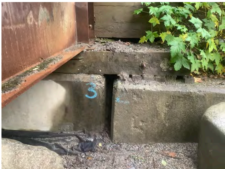
Downstream left bearing
