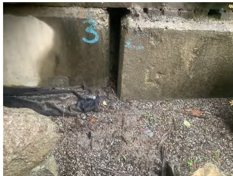
Remedial fill heath blocks
