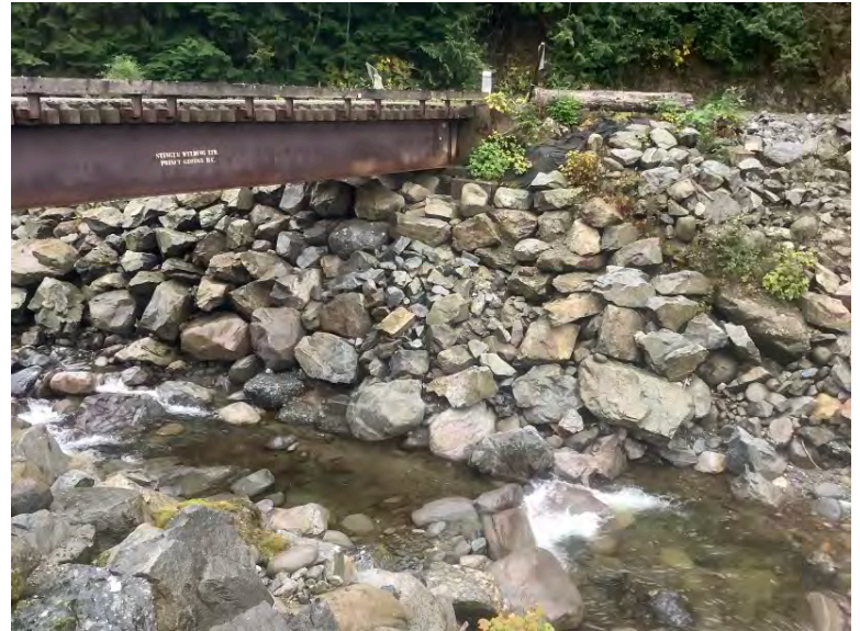
Left Bank Abutment when facing downstream
