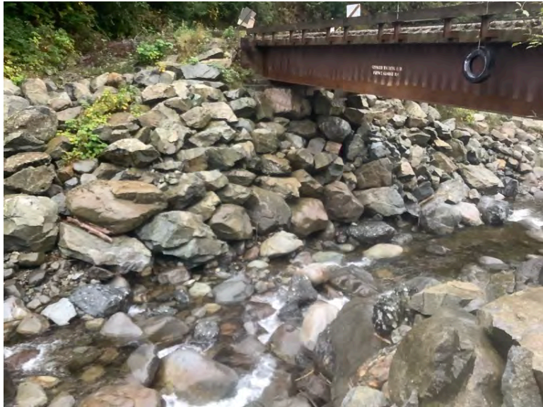
Left Bank Abutment when facing downstream
