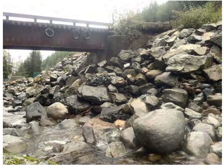
Right Bank Abutment when facing downstream
